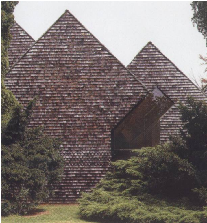
Sinagoga do Jewish Center of The Hamptons - "Gates of the Grove", Easthampton, NY, EUA, 1989 – Norman Jaffe. Fachada lateral. Fonte: MEEK, 1996, p. 227.
