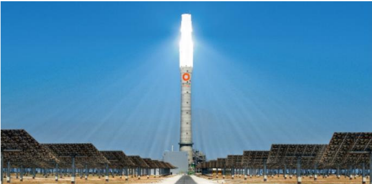
Fig. 13. Gemasolar 140 meter high solar power tower, Seville, Spain (20 MW)
